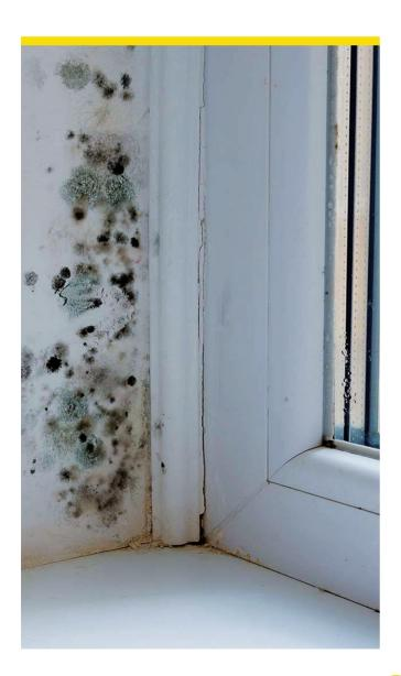
To minimise the risk of condensation it is necessary to drive out the moisture through careful heating and ventilation.
